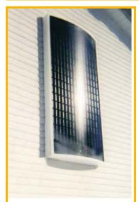
The dimensions, in inches are 44W x 88.5H x 4 thick at sides, 8.5 thick at the center. Rather than being flat, the glazing on the Cansolair panel is rounded so that it wraps around the unit, catching the sun for more hours of the day. You can see this curve in the picture above, and the dimensions below.
